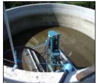
Effluent tank installed below the dairy
