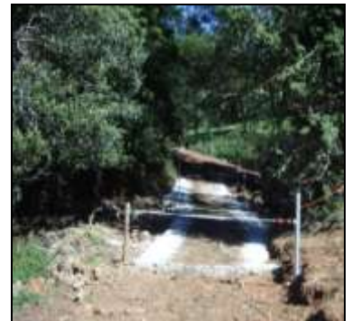
One of five causeways installed.
