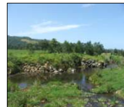
3-yr-old revegetation above 1 of 4 rock structures installed on Fountaindale Creek
